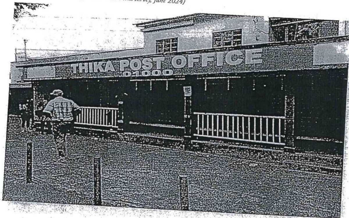
Figure 26: Thika Post Office (Source: Field survey, June 2024)
