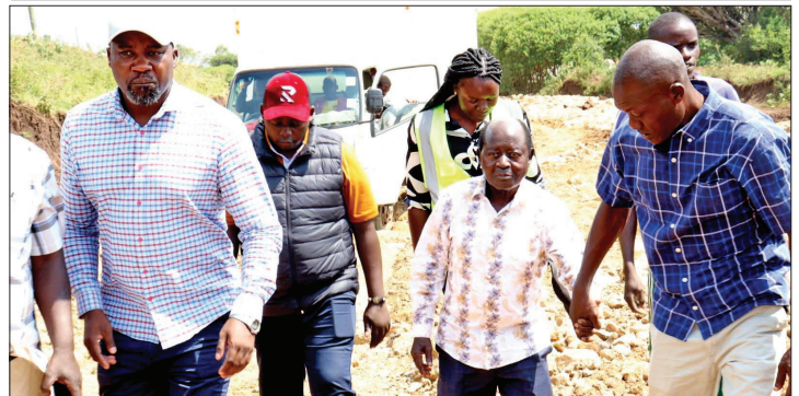
Karachuonyo MP Hon Adipo Okuome (in a white shirt) leads other officers in inspecting ongoing works on Ojijo Ring road in the constituency.
