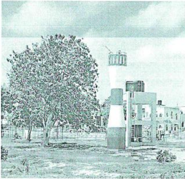
(i) Maintained Vasco rear leading light.
