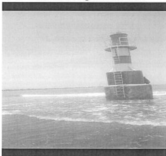
(i) Maintained Malindi front leading Light
