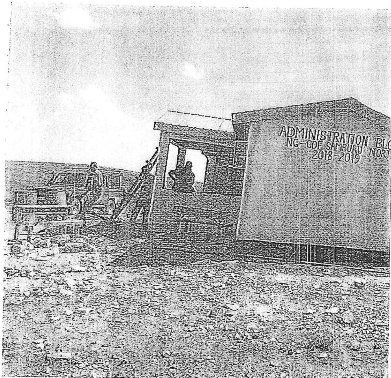
ongoing construction of administration block at Simiti primary school
