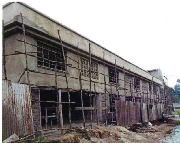
Construction of the KNH-Othaya laundry at KNH
