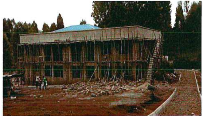
Construction of the KNH-Othaya Kitchen
