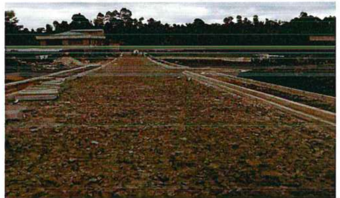
Construction of the KNH-Othaya access and service roads
