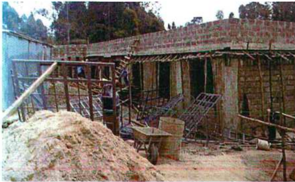
Construction of the KNH-Othaya Mortuary
