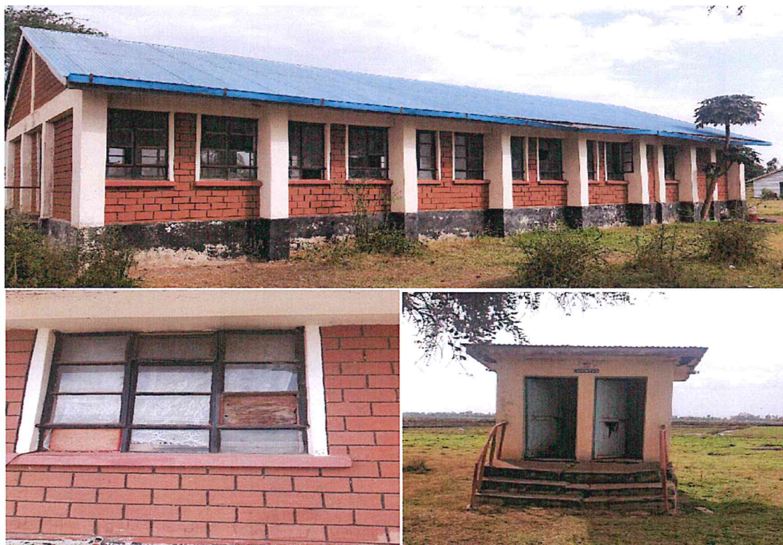
Photos showing broken window panes in the evacuation hall and the status of the ablution block Source: Photos taken by the audit team in February, 2022
