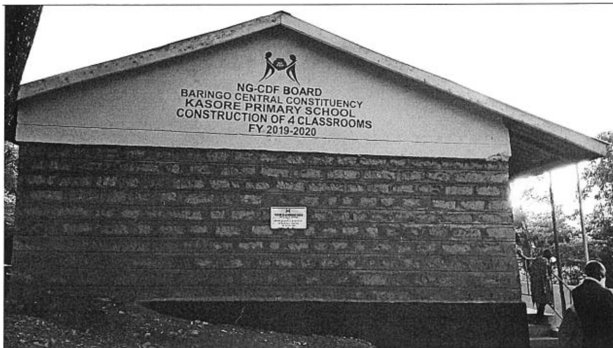
Kasore Primary School Construction Of 4 Classrooms
