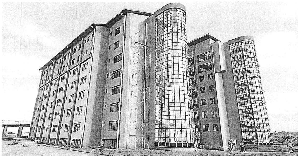
Fig. 20: KAS 7-Storey Hostel building
