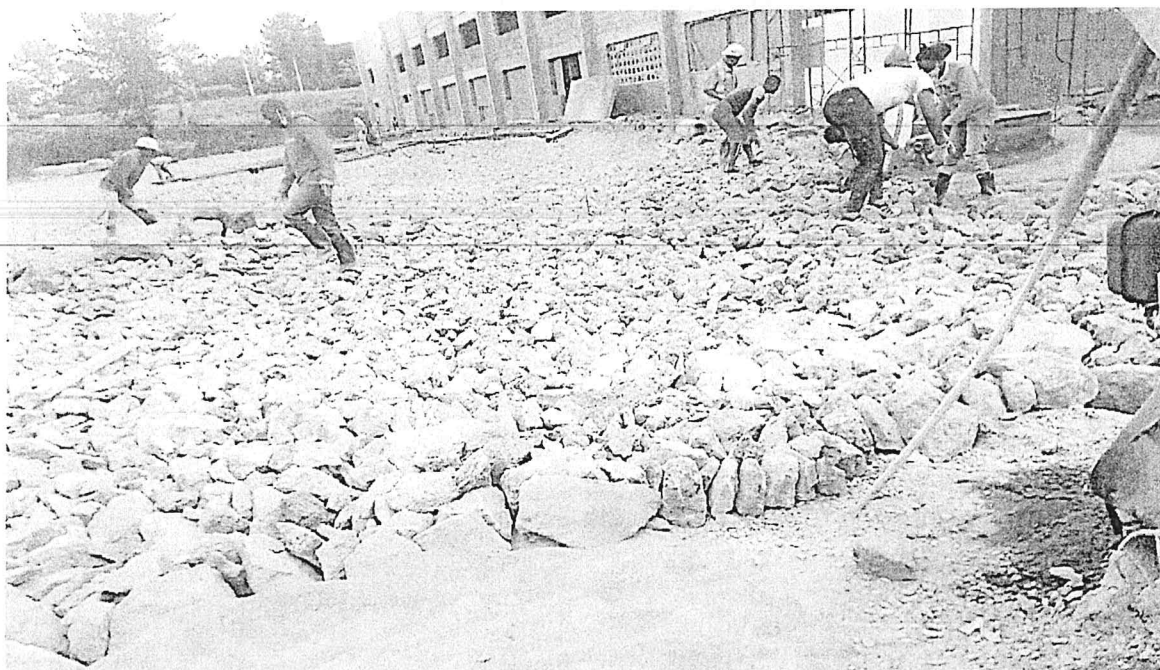
Fig 15: Hard-core hand packing of the Public parking
