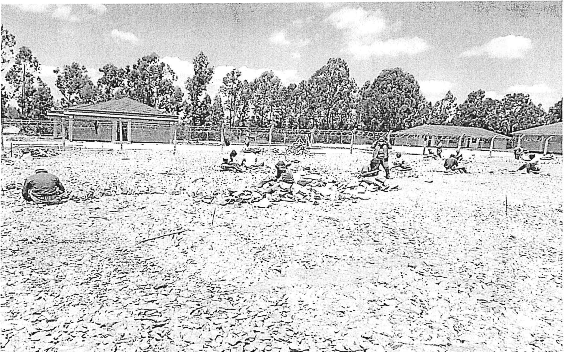
Fig 9: Hardcore hand Packing for main Car Park
