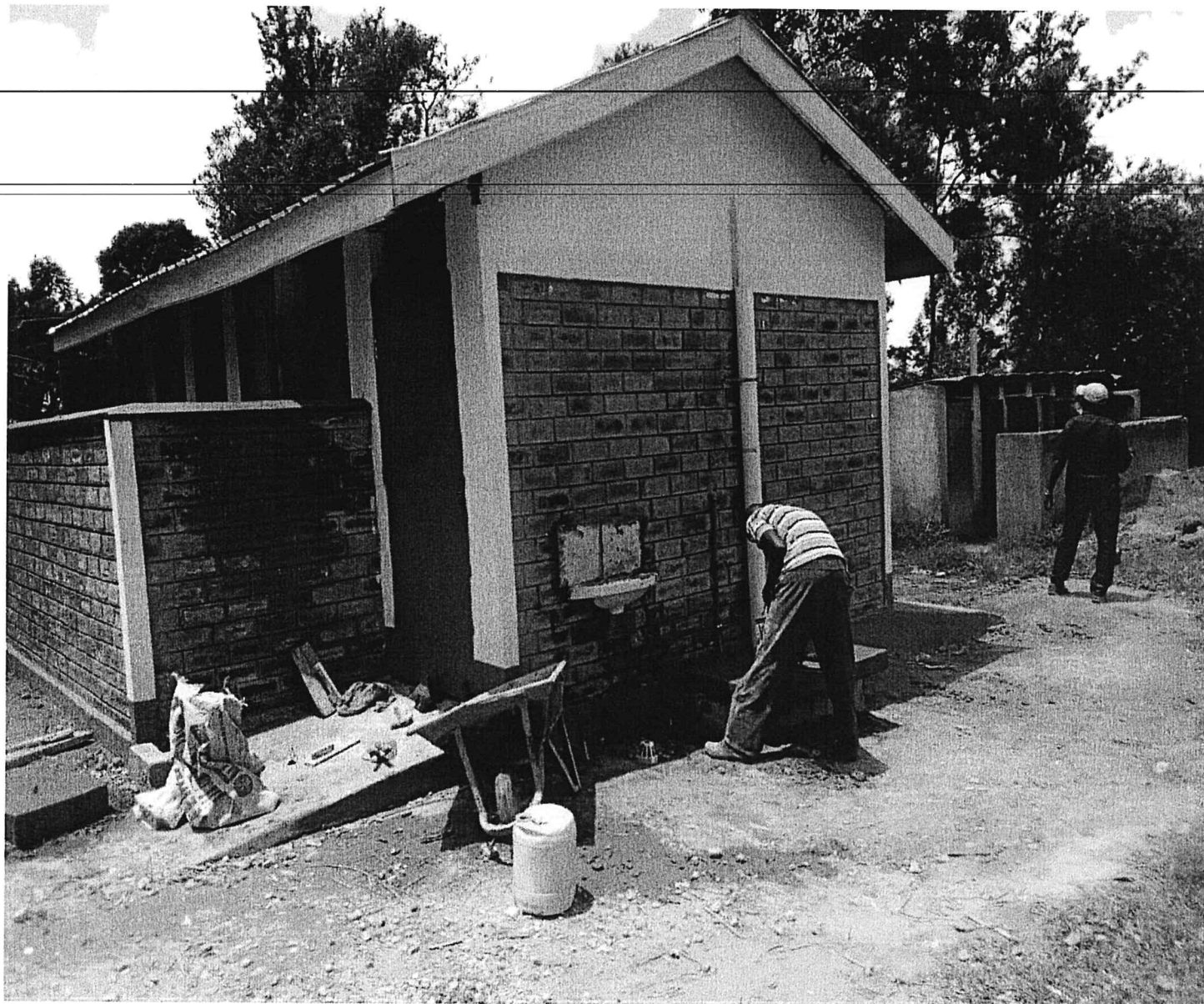
Project Name: Ruambwa Primary school Activity: Construction of a 12-door modern flush toilet with a solar pump water supply.
