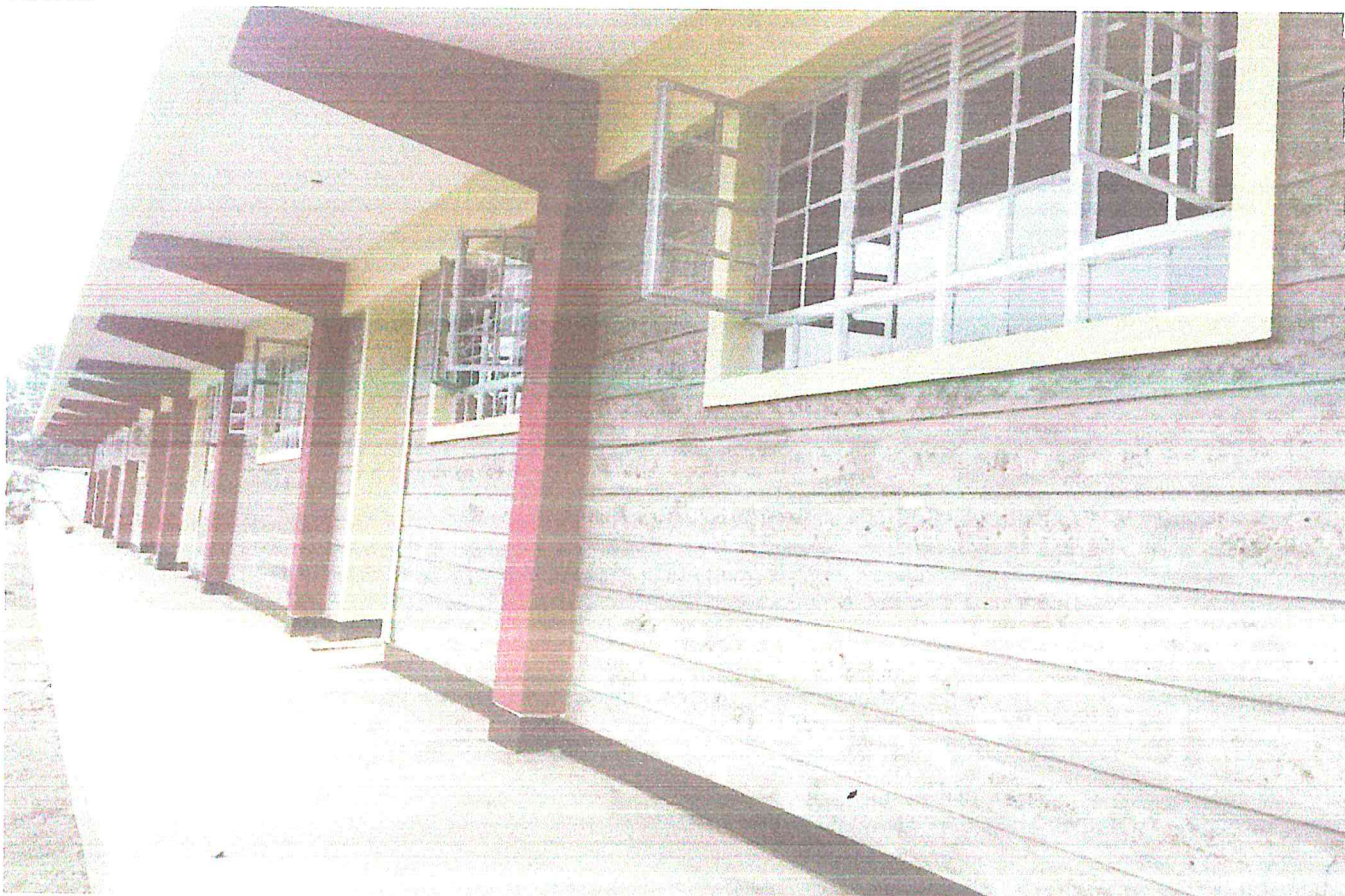
St. Dominic secondary 4 No. classrooms construction
