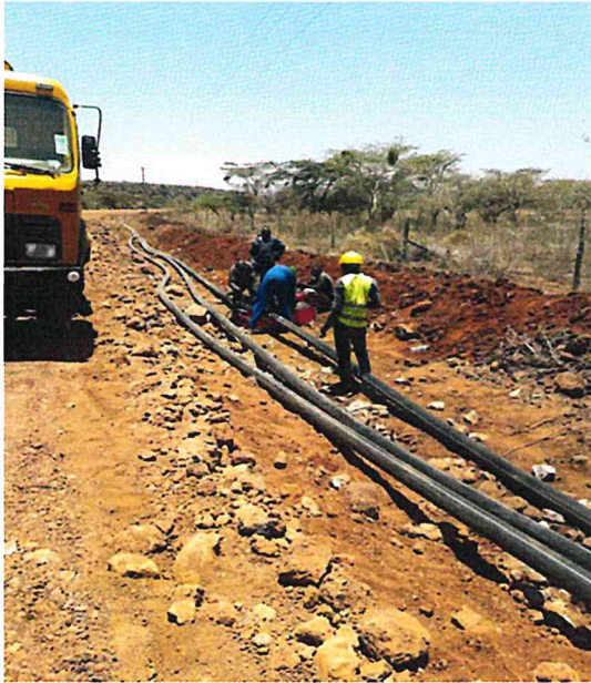
Excavation for laying of the 17 km pipel 1
